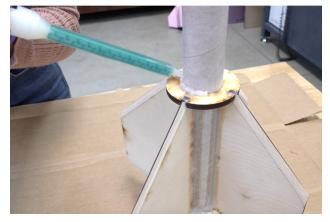
While the assembly is upright glue the forward (top) centering ring in place as well - be sure to apply epoxy over the eye bolt joint as well.
