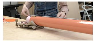
Mark a spot to drill <sup>1</sup>/<sub>8</sub>" aft from your line. This should be in the center of your centering ring, giving the screw something to bite into.
